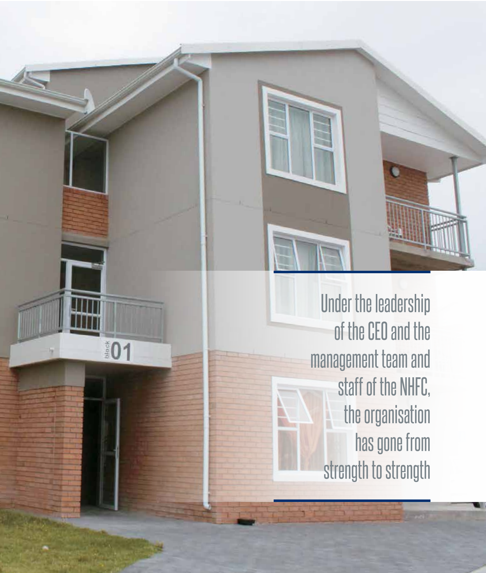
Fairview Link – Port Elizabeth
