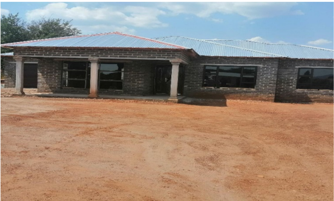
Roofing renovation, Ledig Area in Bojanala District Municipality, North West.
