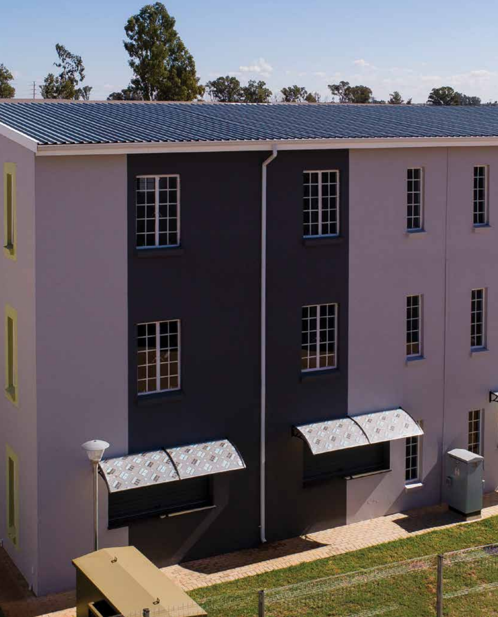
Matlosana project, Klerksdorp, Northwest
