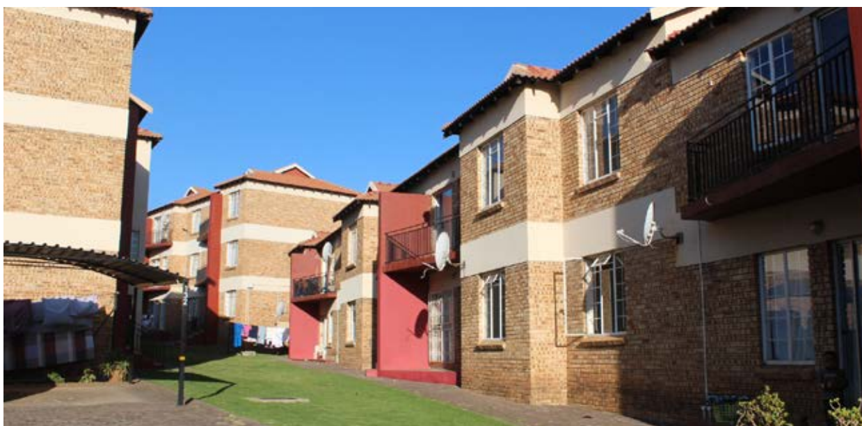
Kyle's Place Project, Gauteng
