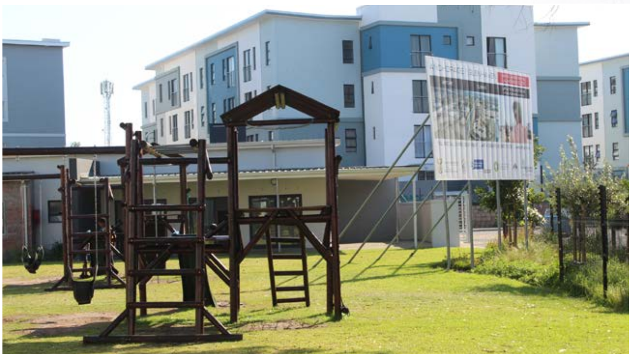
Anchorage Glenhaven Project, Belville, Western Cape
